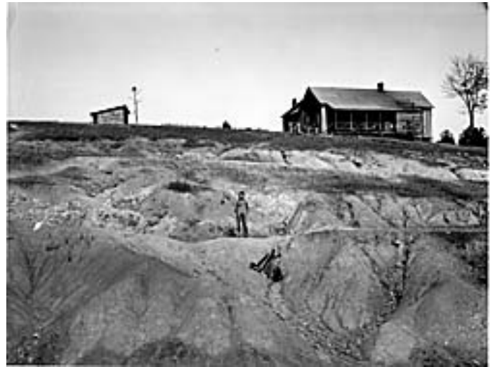
Soil erosion in Alabama
