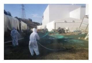
Workers spray adhesive synthetic resin over the ground at the Fukushima Daiichi nuclear power plant. Photo / AP
